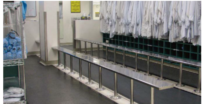
Figure 2: Changing area covered with Dycem CleanZone polymeric floor covering
