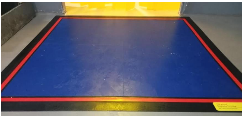
Image 4. Scratch noted in the Dycem Contamination Control Flooring due to rotation of jack lifts
